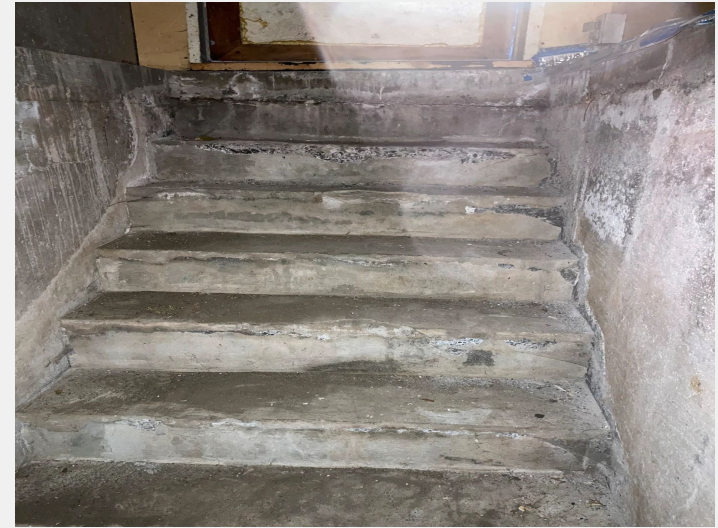
Efflorescence
