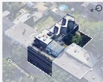
Aerial view of the original building and its backyard expansion.
