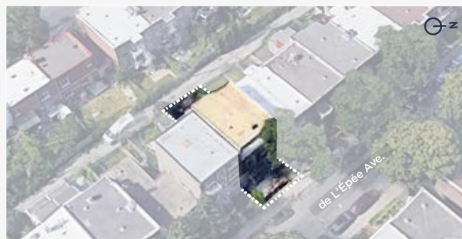
Aerial view with the new storey constructed to the building alignment.
