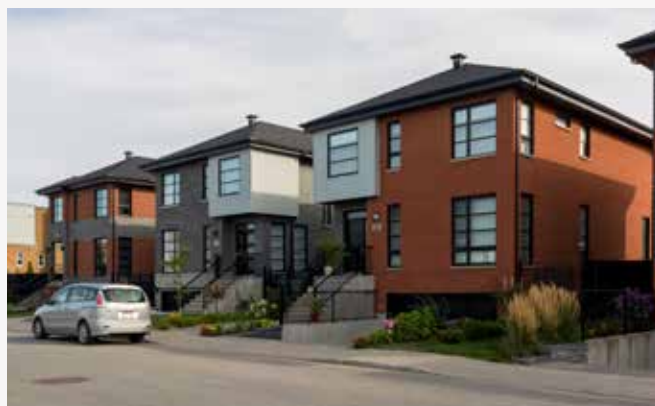
Detached single-family homes comprise most of the low-density group constructed during the first phase.
