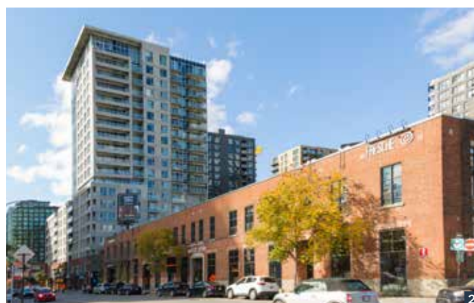
Buildings of different volumes, seen from rue Wellington.
