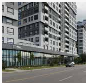
View of the articulation of volumes and commercial windows from boulevard Newman.
