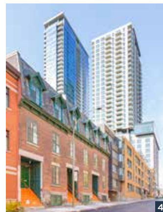
Tours Marriott, including accommodations and residences.
