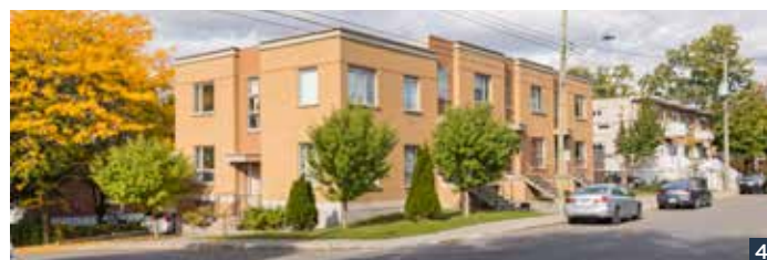
Newly constructed group of townhouses.
