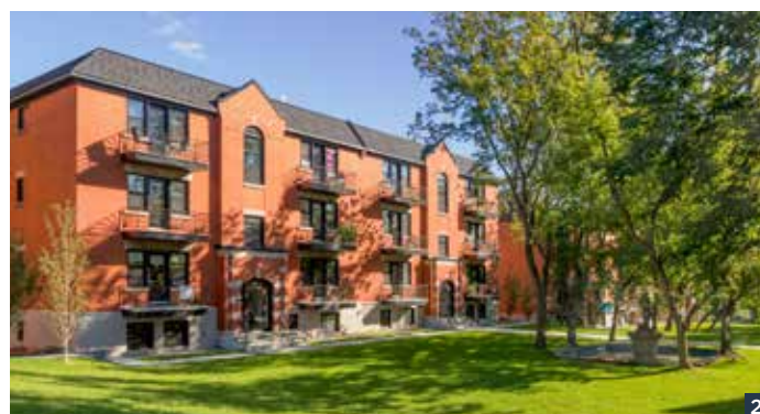
Jardins des Saules, a group of multi-unit buildings organized around a courtyard.
