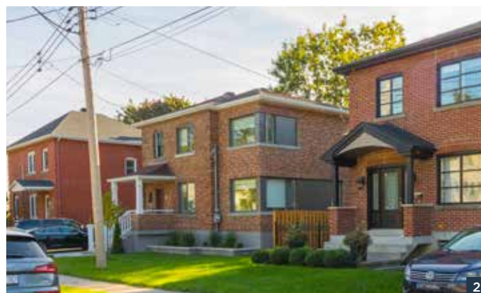
Side expansion integrating with the architectural style of the area.
