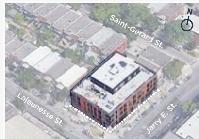
Aerial view of the mixed-use, multi-unit building extending to the end of a block, occupying its entire lot.
